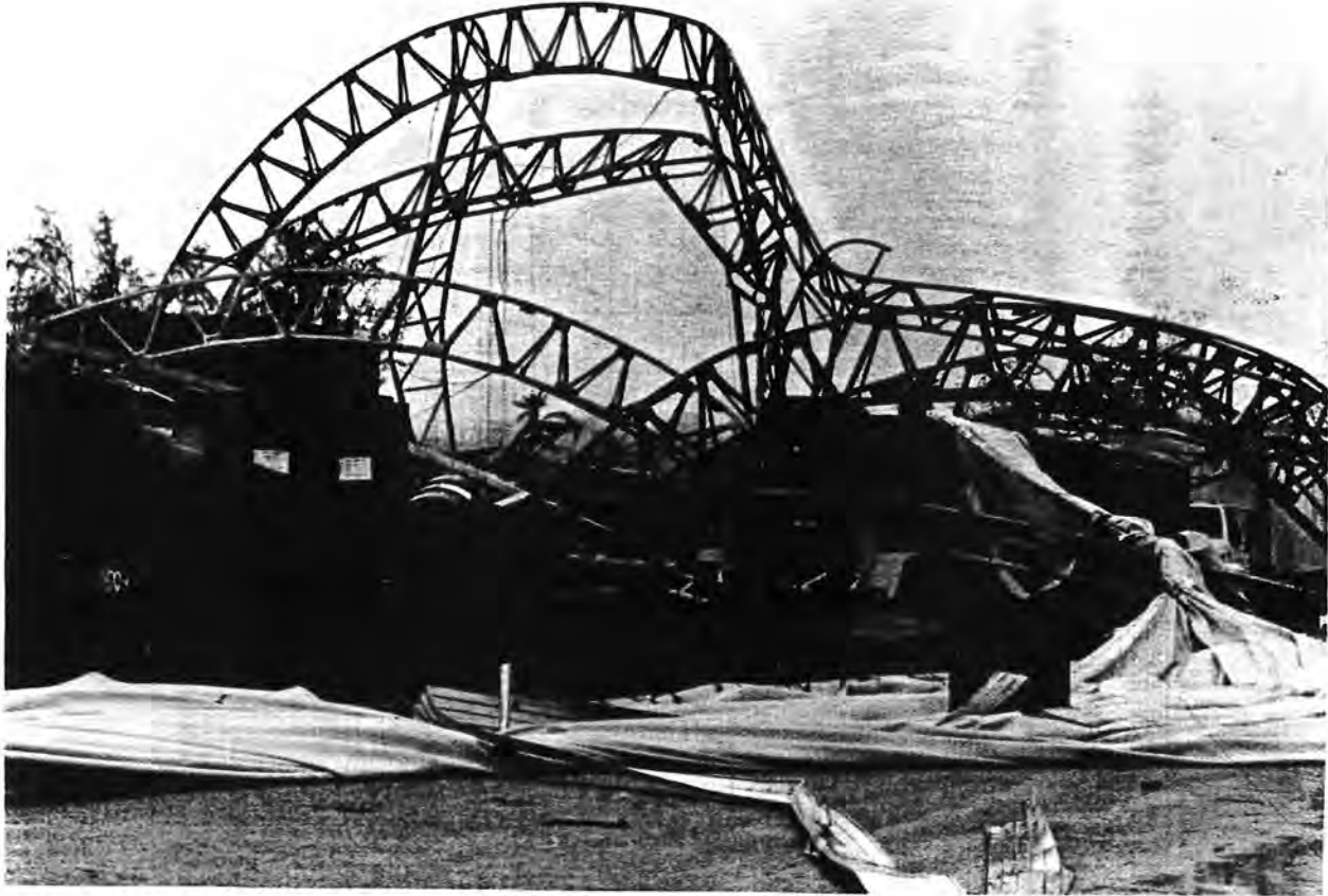
Figure 17. The steel girders of this temporary warehouse on Naval Station, Guam, were twisted by the high winds and collapsed during Russ's passage.
